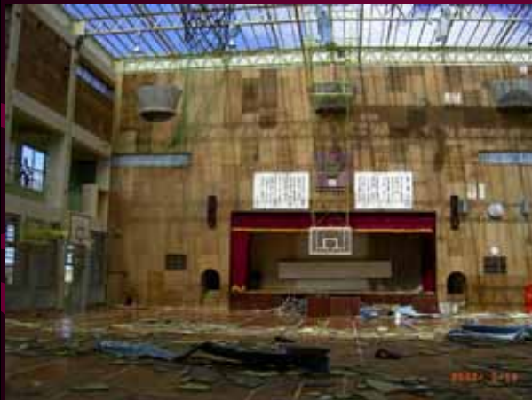
Damage to a roof of a gymnasium
