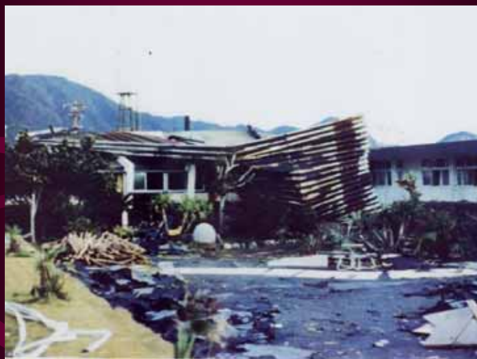
Steel roof sheet flew from upstream (Typhoon 7513)
