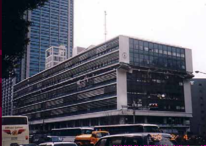
KOBE EARTHQUAKE, Jan. 17, 1995
