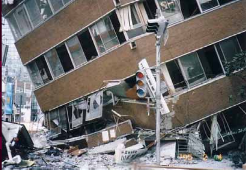
KOBE EARTHQUAKE, Jan. 17, 1995
