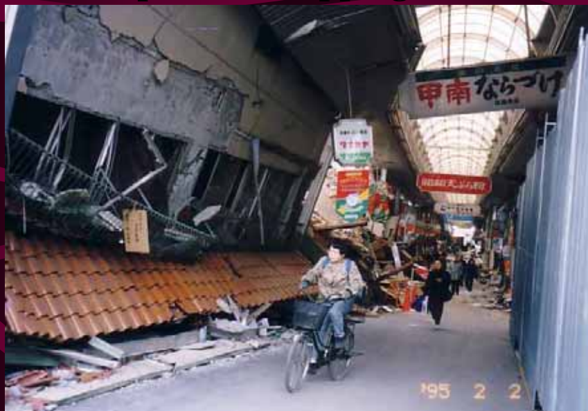
KOBE EARTHQUAKE, Jan. 17, 1995
