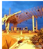
Fig. 4 Highway entrance roof
