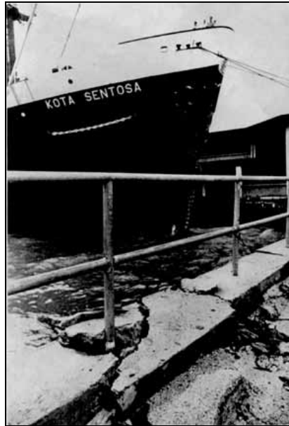
Figure 27: Damage to berth caused by SS Kota Sentosa (after HKO)
