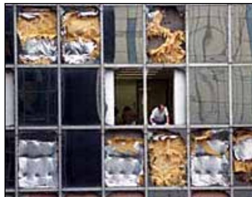
Figure 4: Aftermath of Typhoon York - Left: Damaged curtain walls of Central Plaza (striped building) and Immigration Tower; Right: Close-up of damage to Immigration Tower (after van der Woning)
