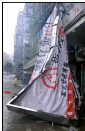
Figure 6: Damaged signboards caused by Typhoon York (after van der Woning)
