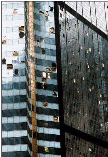
Figure 4: Aftermath of Typhoon York - Left: Damaged curtain walls of Central Plaza (striped building) and Immigration Tower; Right: Close-up of damage to Immigration Tower (after van der Woning)
