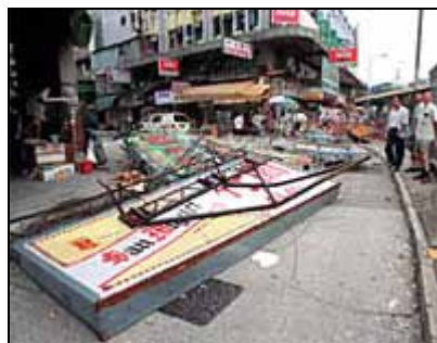
Figure 6: Damaged signboards caused by Typhoon York (after van der Woning)
