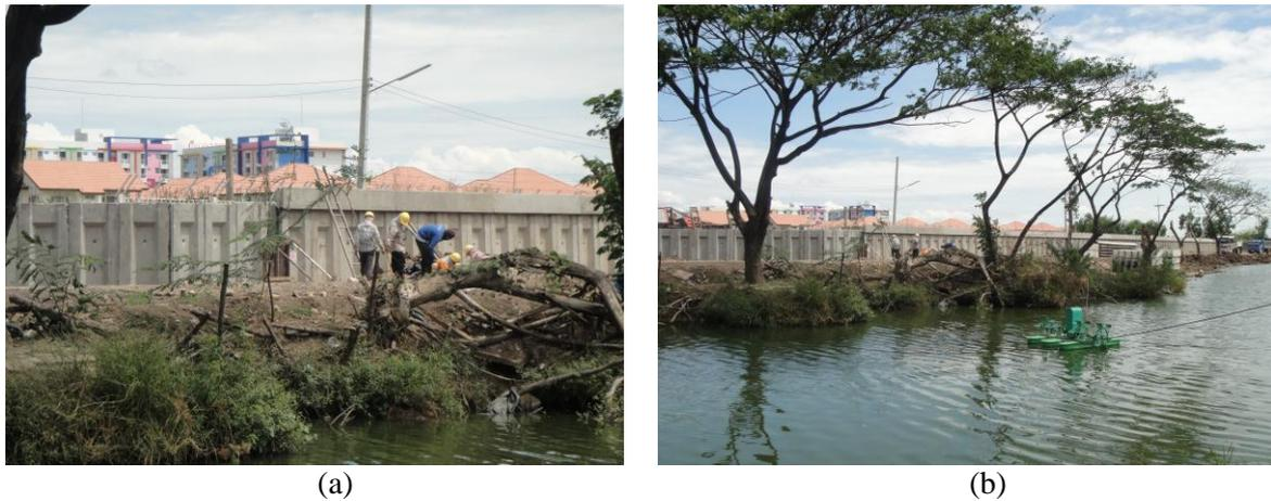
Figure 13. (a-b) Examples of flood prevention of Thammasat University, Rangsit Campus by new concrete-sheet-pile and soil dam in year 2012.
