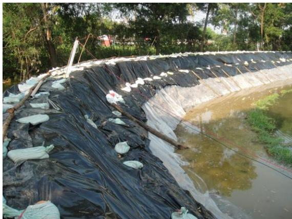
Figure 12. Examples of flood prevention of Thammasat University, Rangsit Campus by old soil dam in year 2011
