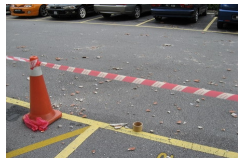
Figure 2d: Flying Debris of Roof Tile
