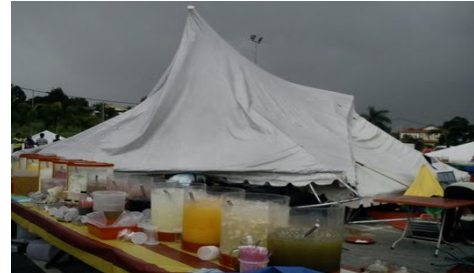
Figure 1d: Canopy Collapse
