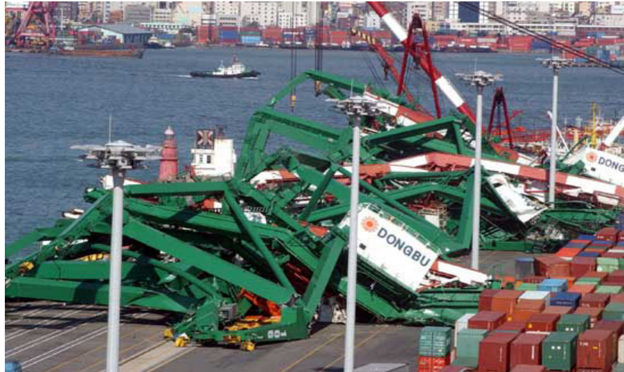
Fig. 2.1 Gantry Cranes Overturned by Typhoon Maemi
